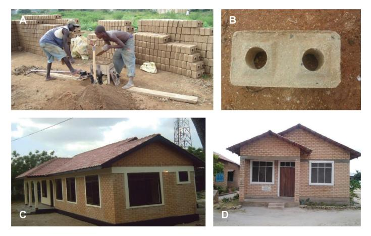
Figure 3. (A) Fabrication of interlocking soil-cement blocks; (B) Finished soil-cement block; (C) Construction made in 2000 by the NHBRA using interlocking soil-cement blocks in Tanzania; and (D) Example of a house built by the NHBRA in Chamazi, Dar es Salam. Source: NHBRA<sup>43</sup>
